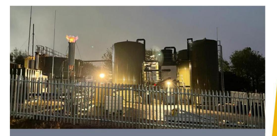
"This picture shows the biomethane burner of our effluent plant in action which powers the CPH (combined heat and power) engine that generates up to 65kW of electricity per hour."
